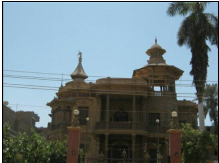
Pl.2. The Northern facade of 'Abdelmagīd Seif el Naṣr palace. The Researcher
