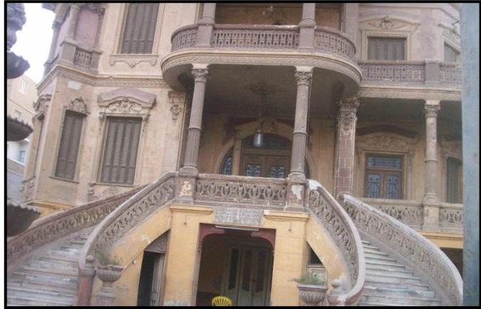
Pl.8. The double staircase leading to the main entrance of 'Abdelmagīd Seif el Naşr. palace. The Researcher
